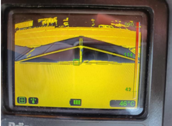
Figure 6: Thermal imaging surrounding roof area 1st September 2022 showing temperatures exceeding 46 °C on surrounding areas
